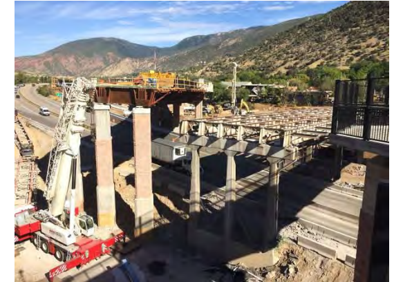
Denver Metro West I-70 Bridges
