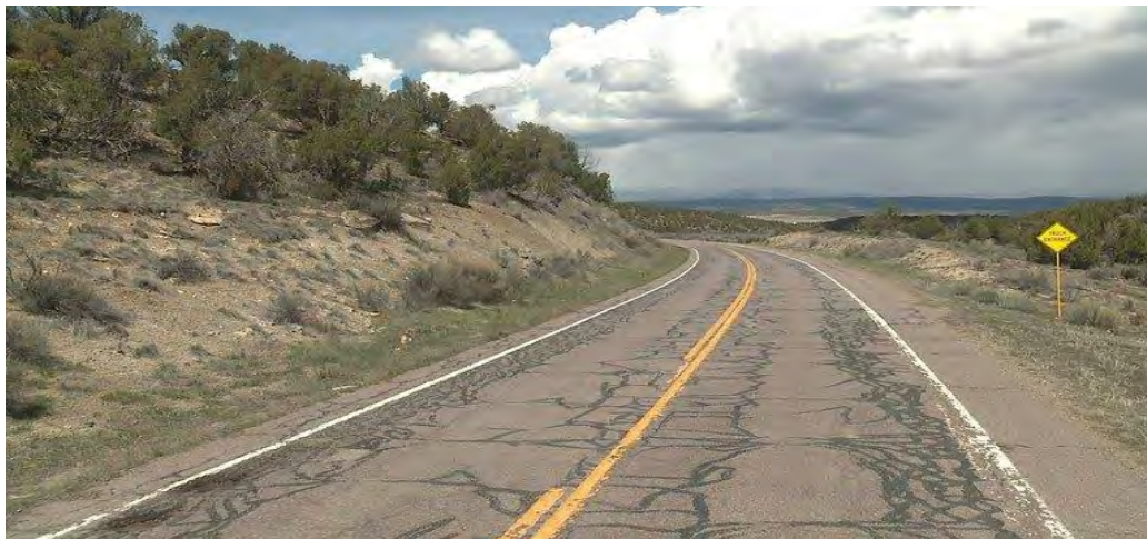
Shovel ready rural road rehabilitation and maintenance in tourism corridors and scenic byways
