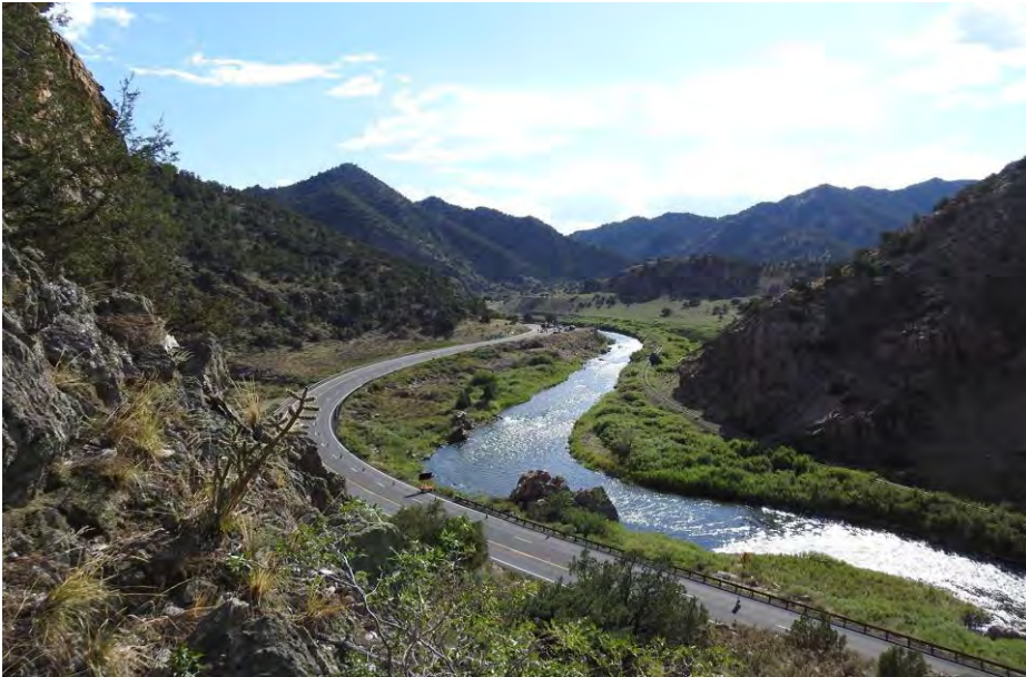
Surface treatment, bridge rehabilitation, and guardrail improvement project on US 50 in Fremont county
